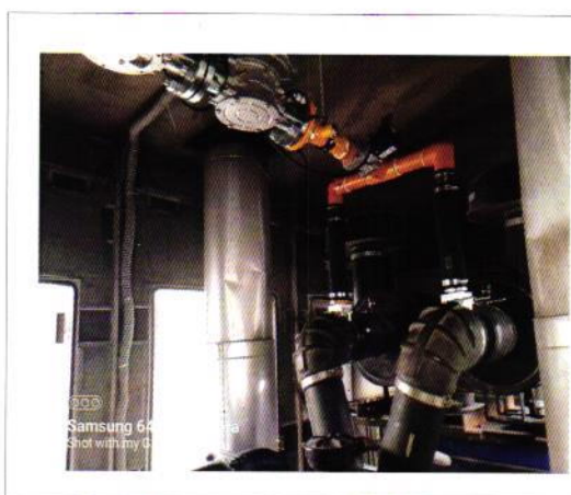
Dual Fuel System in DG Set
